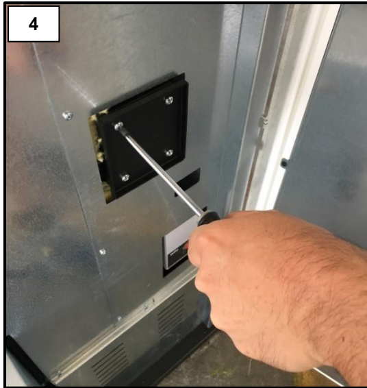
Remove the “extractor flue gas pass inspection front plate” by unscrewing the 4 screws (figure 4). Using the ash vacuum, vacuum the deposit inside (figure 5).
