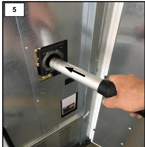
Remove the “extractor flue gas pass inspection front plate” by unscrewing the 4 screws (figure 4). Using the ash vacuum, vacuum the deposit inside (figure 5).
